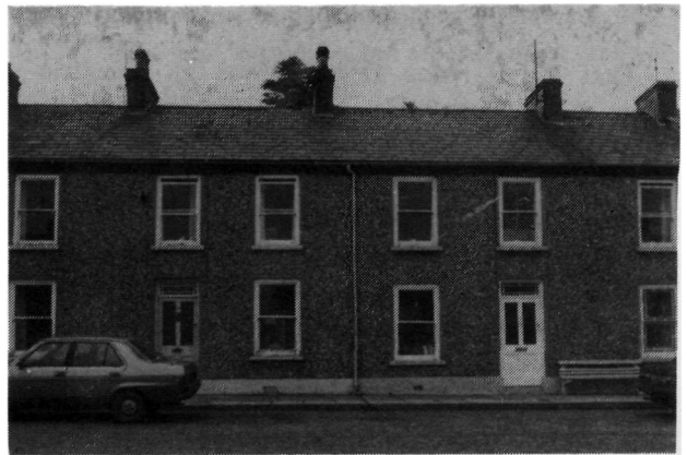
Dr. MacDermott's house and the "dispensary" Church Street
