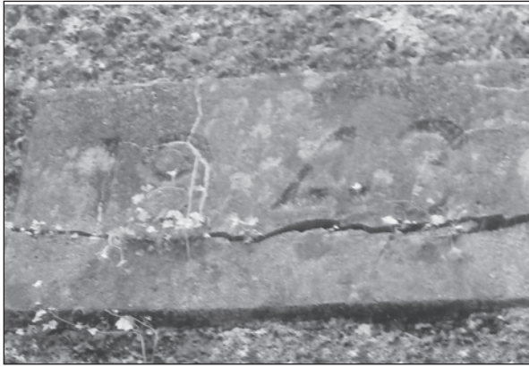
Plaque recording the last major renovation in 1943.
