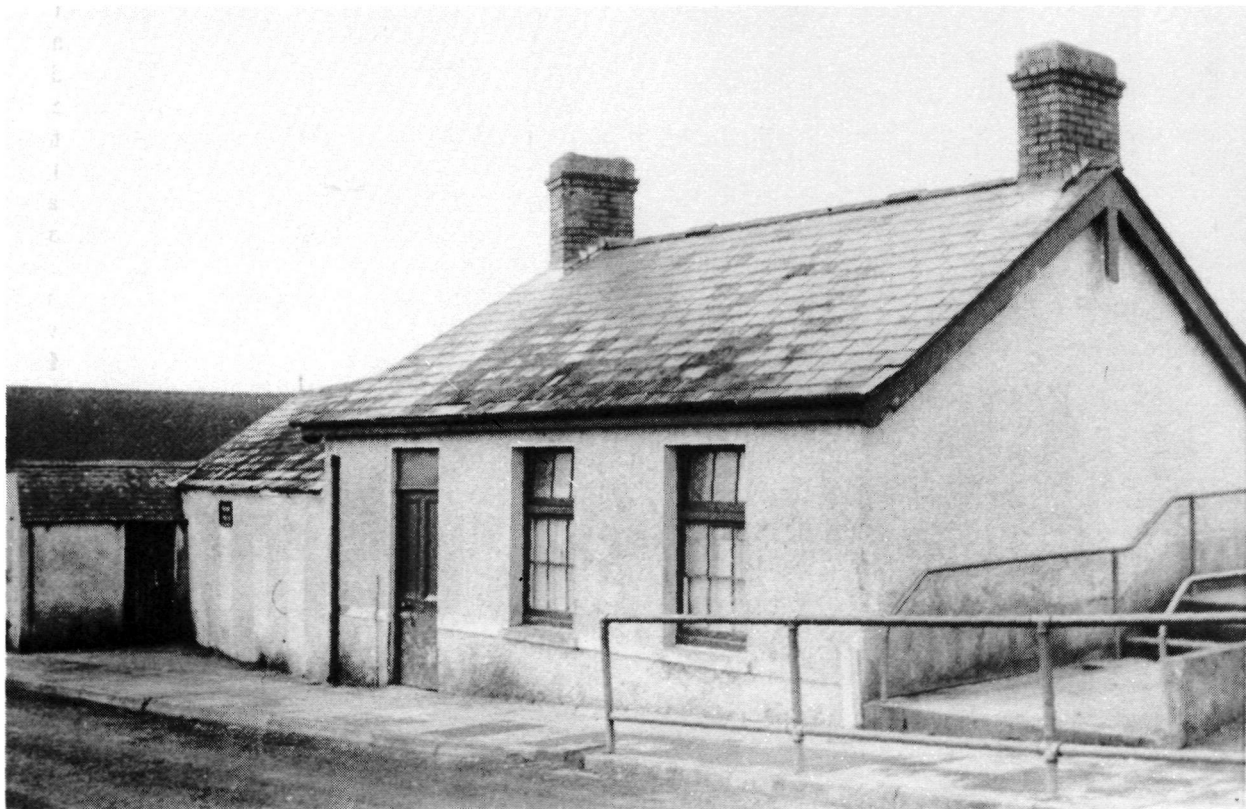
The old Schoolhouse shortly before demolition.
