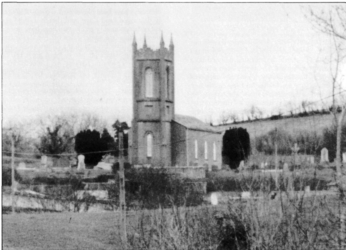
Donaghmore Church suffered severe damage.
