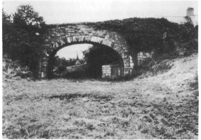
Kilmonaghan Road Bridge, South of Jerrettspass
