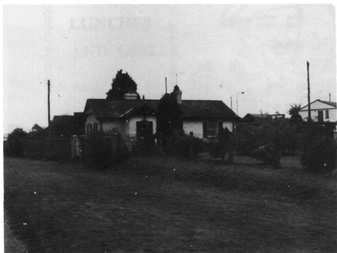
Stationmaster's house at Loughgilly
