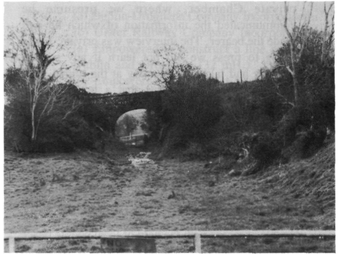
Bridge North of Ballydougherty
