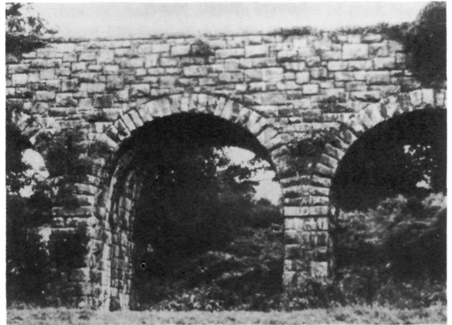
Tripe Arch 'under bridge' at Jerrettspass
