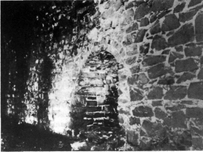
Interior of tunnel showing recesses
