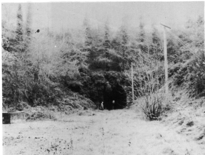
Entrance to Loughgilly Tunnel (exit is also visible)
