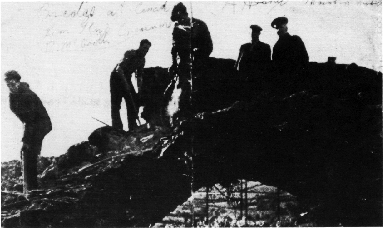
Workmen demolishing 'The far 'Pass bridge' 1951. In the picture is Constable Gethins.
