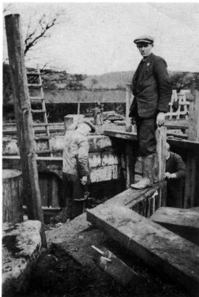
Joe Monaghan supervising repairs to Crothers' locks.
