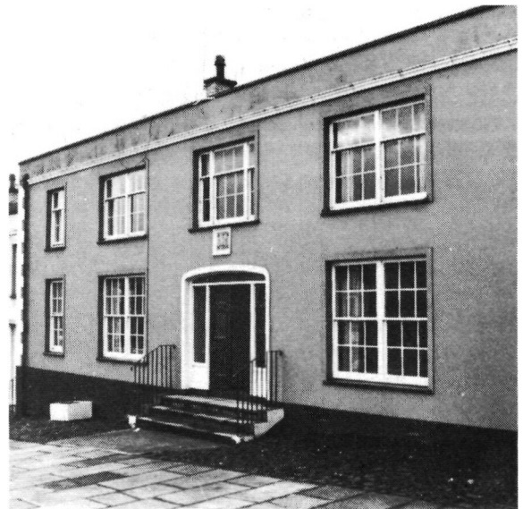
The site of Tandragee Courthouse.
