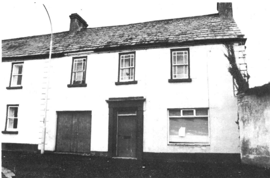
Poyntzpass Courthouse to-day.
