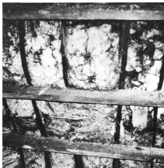
Sods to the underside of a thatched roof.
