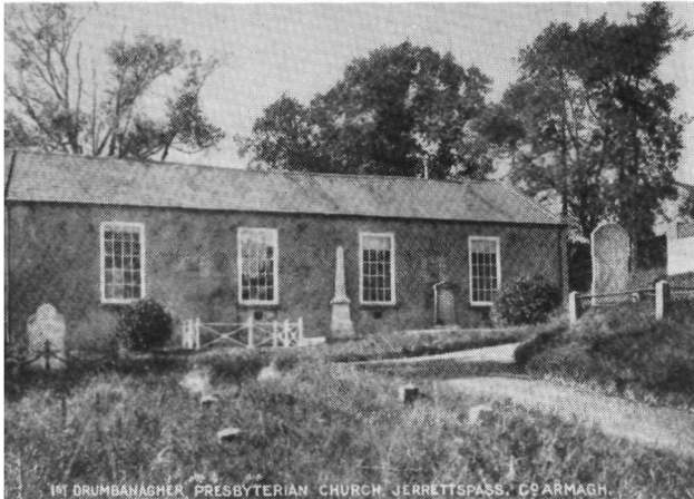
1st Drumbanagher Presbyterian Church, Jerrettspass
