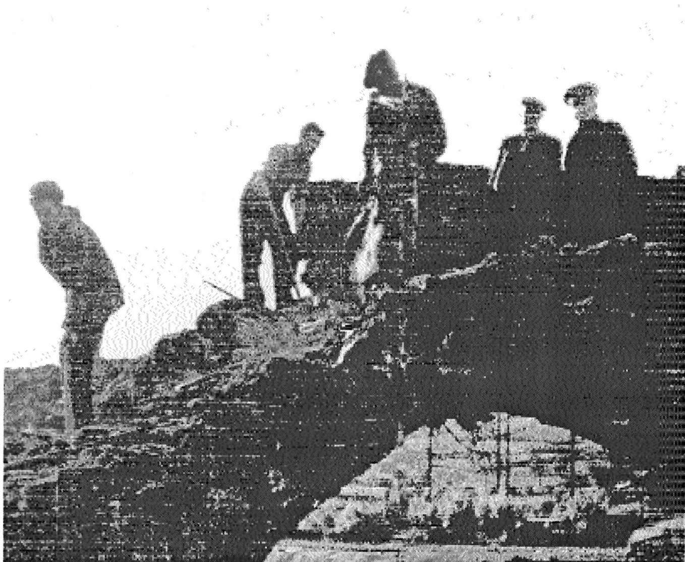
Workmen demolishing the Far Pass bridge 1951 while Constable Gethins looks on.
