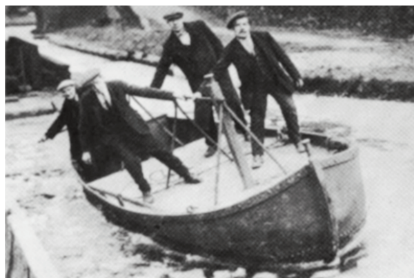
An 'Ice-Breaker' - Similar to one used on the Newry Canal
