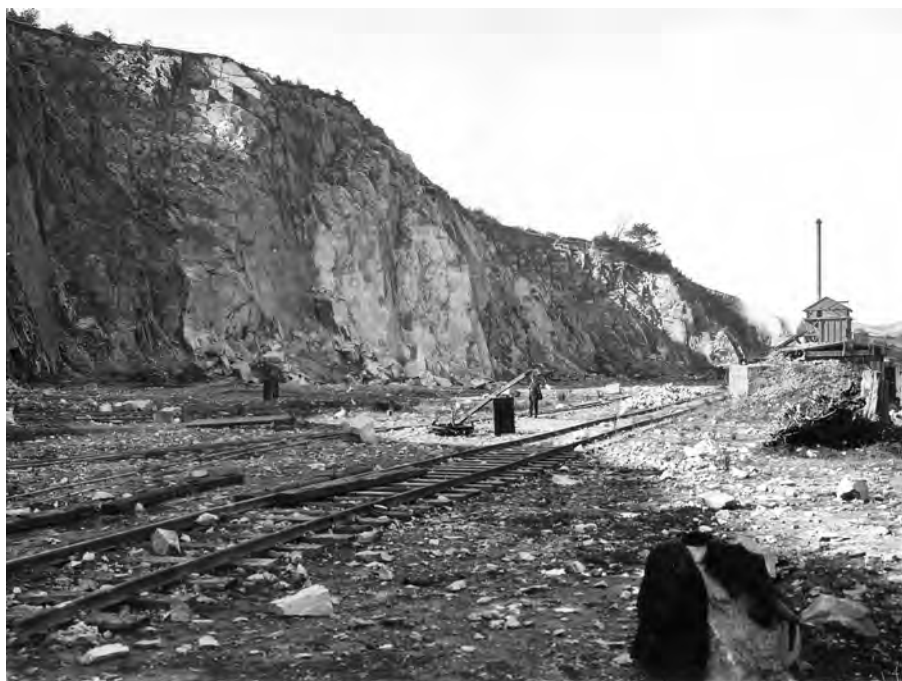
Goragwood Quarry after a blast.
