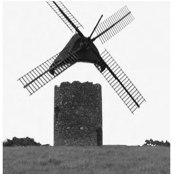
***Replacing the cap!!!***
