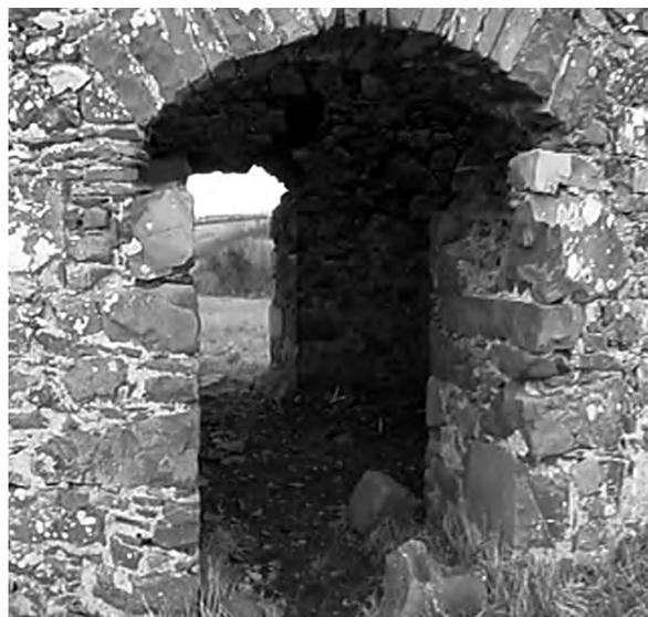
Our windmill stump is over 21 feet in height and 17 feet in diameter at its base. The walls are 3 foot 9 inches thick and there are two doors and one window with two narrow apertures above the doors. I would calculate overall height complete with cap at about 30 feet compared to 33 feet at Ballycopeland. Our diameter is 17 feet at the base, Ballycopeland 22<sup>c</sup> feet. The walls of the mill slope inward and the slope is known as the batter.
