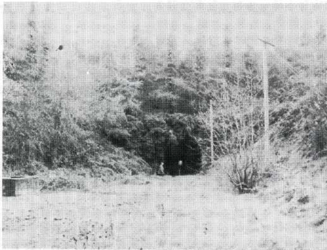
Entrance to Loughgilly Tunnel (exit is also visible)
