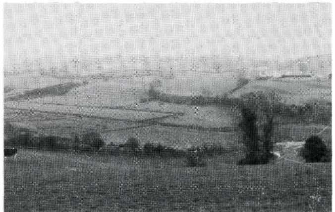
Embankment across Loughilly Bog
