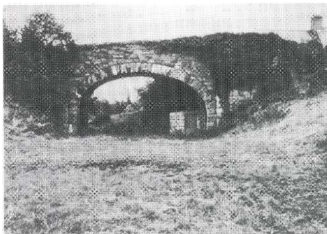
Kilmonaghan Road Bridge, South of Jerrettspass
